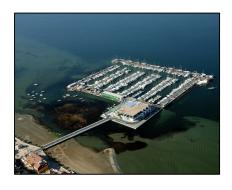
This complete upgrade has 4 lines of 100m of metal frame dock with a gangway.
